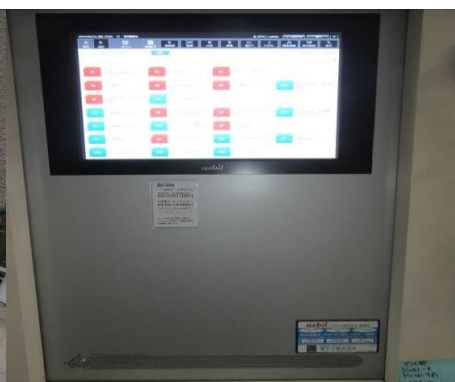
Repaired the heating and air-conditioning system
