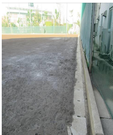
Cleaned the drainage of the school ground
