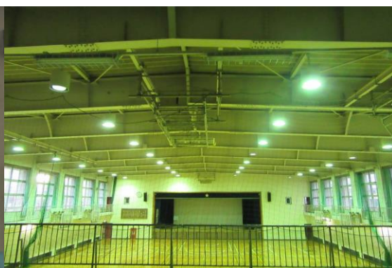
Replaced 32 gymnasium lamps
