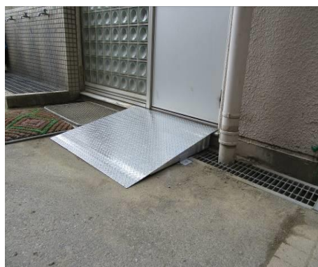
Replaced the ramp
