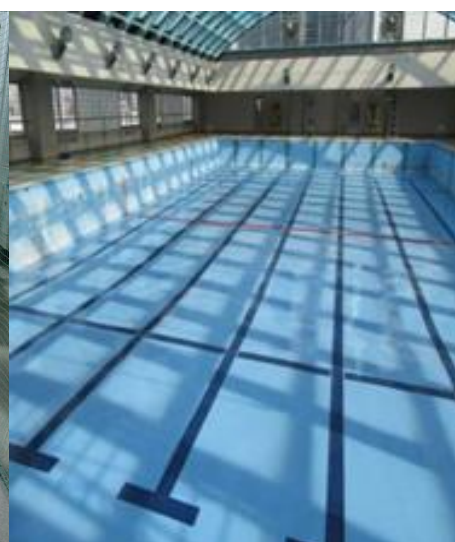
Painted the bottom surface of the swimming pool
